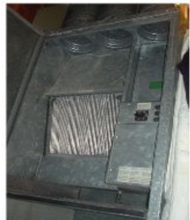
Fig.E.11: De warmtewisselaar in de "Heatkeeper"
